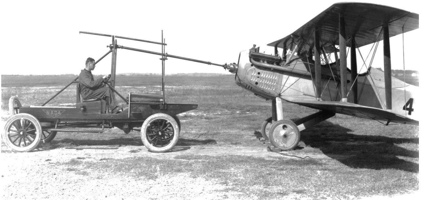
A NACA Hucks Starter with a Vought VE-7 at the Langley Research Center, 1926
